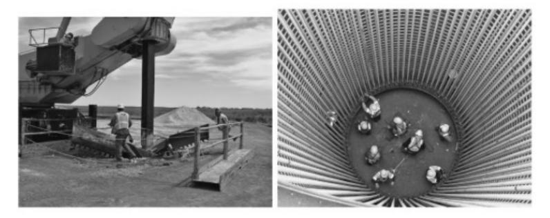
FIGURE 6.22 Pier foundation, concentric cans, for 3-MW wind turbine. Right: bolt rods are in place and starting to attach rebar.
