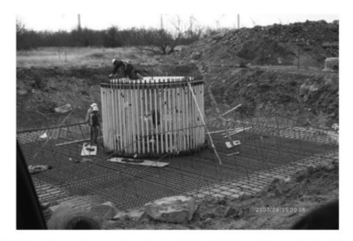
FIGURE 6.20 Placing rebar for pad foundation for 2-MW wind turbine. Finished pad required 32 metric tons of rebar and 270 cubic meters of concrete.
