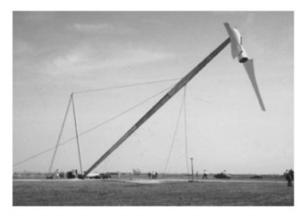
FIGURE 6.19 International Wind Systems 300-kW system on 49-m pole tower with guy wires and gin pole.
