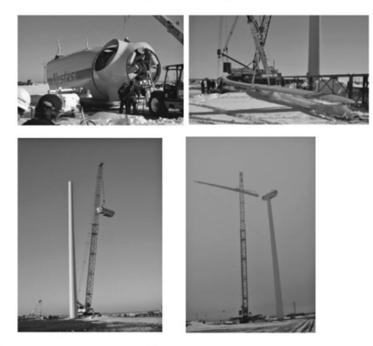
FIGURE 6.23 Photos showing stages of erection of 3-MW wind turbine.
