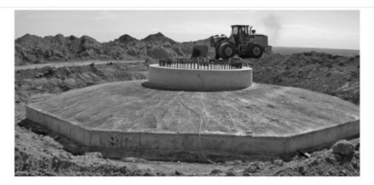
FIGURE 6.21 Finished pad foundation for 2.3-MW wind turbine. Note copper wire for grounding.
